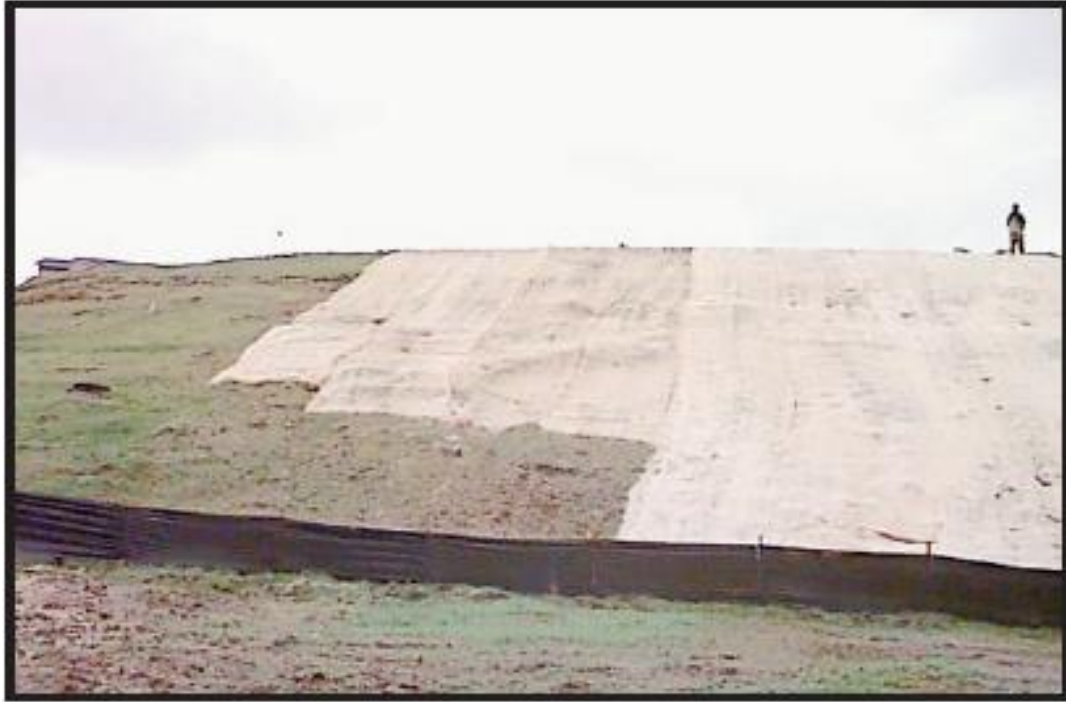
Plate 3 – Coconut matting and silt fence (Source: CIRIA, 2006 10 )
